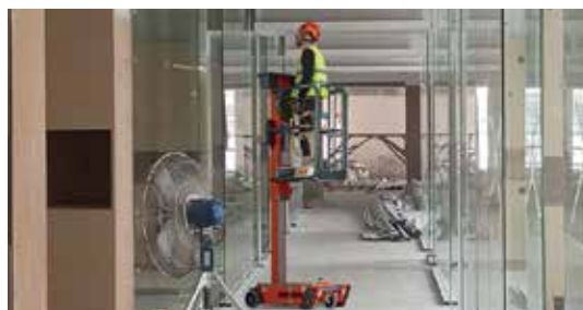
Wider adoption of low level platforms requires 'method change' away from ladders, podiums, small towers or even larger self-propelled lifts' as these typical jobs show - some in the old blue Power Towers colour.
