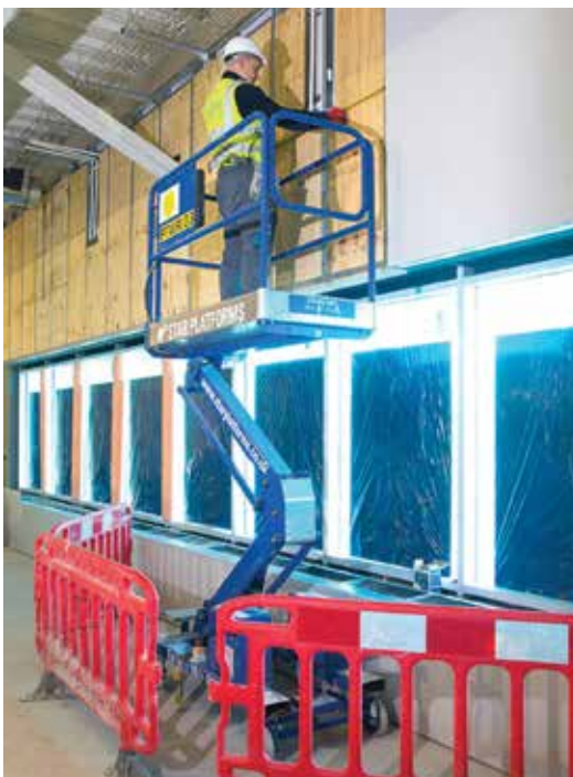
Wider adoption of low level platforms requires 'method change' away from ladders, podiums, small towers or even larger self-propelled lifts' as these typical jobs show - some in the old blue Power Towers colour.
